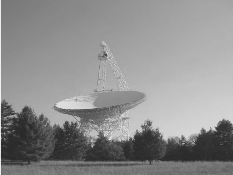
FIGURE 15.2. The Robert C. Byrd Green Bank Telescope of the NRAO in Green Bank WV. This beautiful 330-ft diameter (100-m) dish replaced the old 300-ft that collapsed under its own weight in 1988. The unipod design is meant to reduce unwanted reflections of radio signals from steel beams in the support structure holding up a secondary mirror that then reflects the radio waves to a focus behind the main dish. (Author's photo.)
