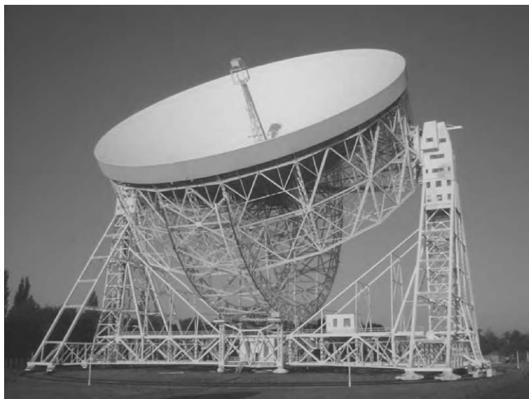
FIGURE 1.2. The 250-ft diameter radio telescope at the Jodrell Bank Observatory in England. At the top of the 60 ft high mast in the center of the dish a box houses electronic amplifiers attached to a small antenna mounted just beneath the box at the focus of the telescope. The amplified signal is then fed down to a laboratory at ground level or, in the days that I was using the dish, to our lab in the tower at the right. This image is of the upgraded version known as the Lovell telescope. The version we used in the early 1960s had only one stabilizing girder carrying much of the weight and the surface was not as carefully constructed. (Photo courtesy of Nuffield Radio Astronomy Laboratories, University of Manchester.)
