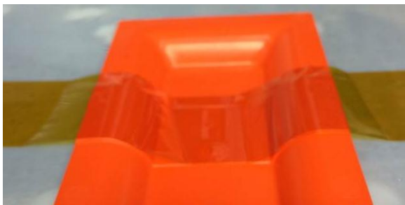
✓ Figure 4 (Tape fully seated on insulator)
