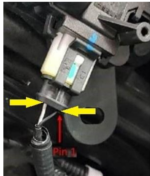
✗ Figure 3 – Incorrect wire position
