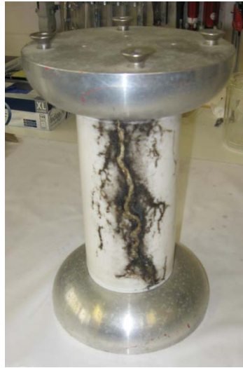
Fig. 15: Tracking caused by water leak across a 35 kV insulator
