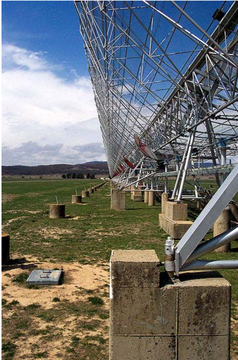
A cylindrical paraboloid antenna.
