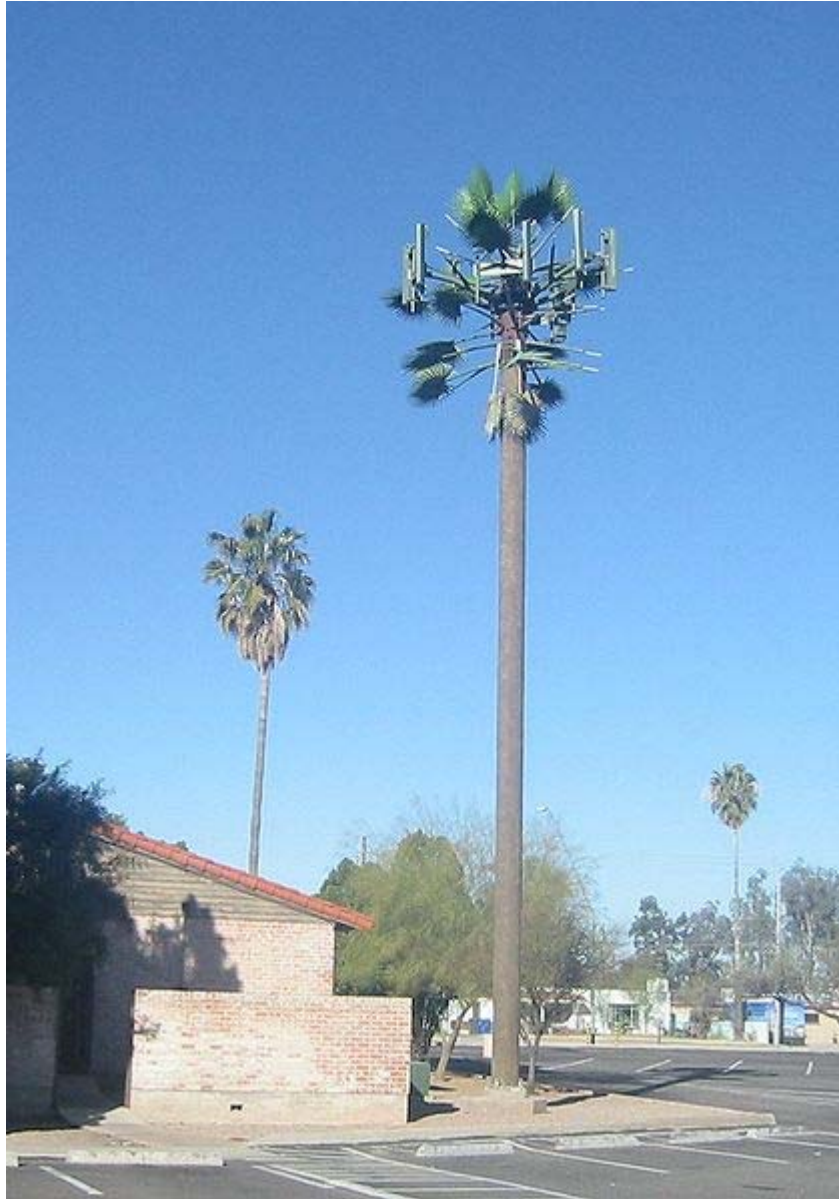
Telephone site concealed as a palm tree.
