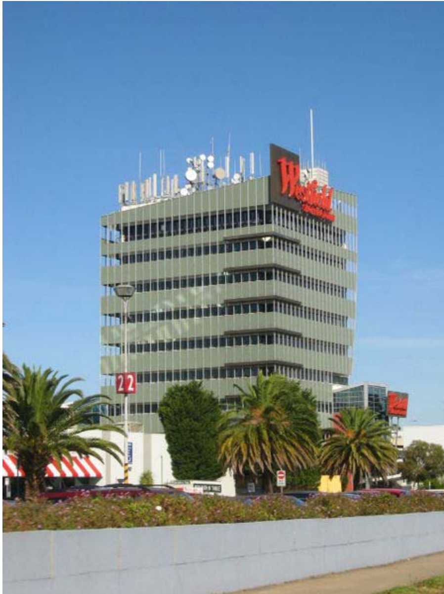
A building rooftop supporting numerous dish and sectored mobile telecommunications antennas (Doncaster, Victoria, Australia).
