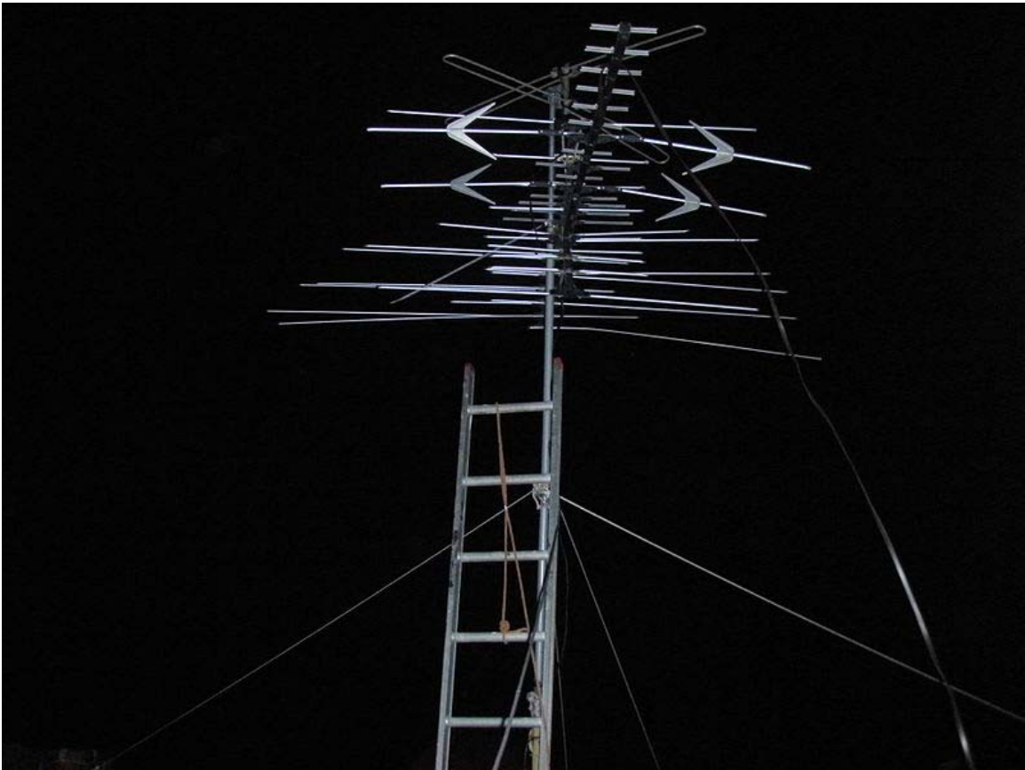
A Winegard HD-7084P 68 element VHF/UHF aerial antenna
