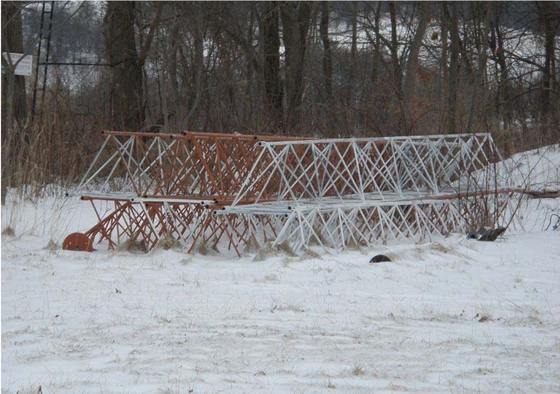
A dismantled radio mast in sections
