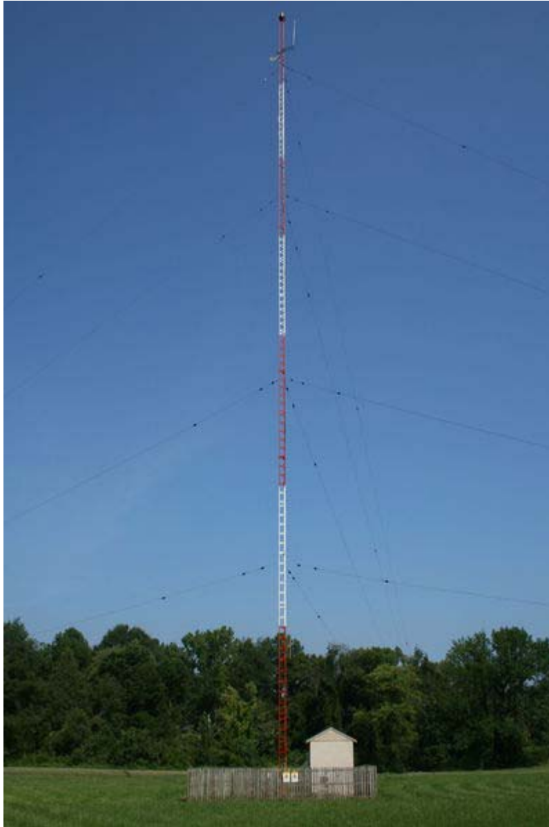
A vertical mast radiator, Chapel Hill, North Carolina
