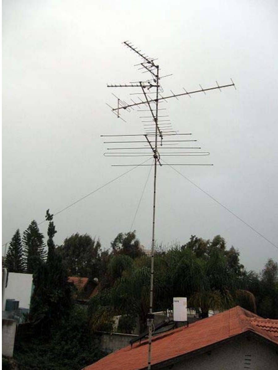
Rooftop directional antennas, typical for use at VHF and UHF frequencies
