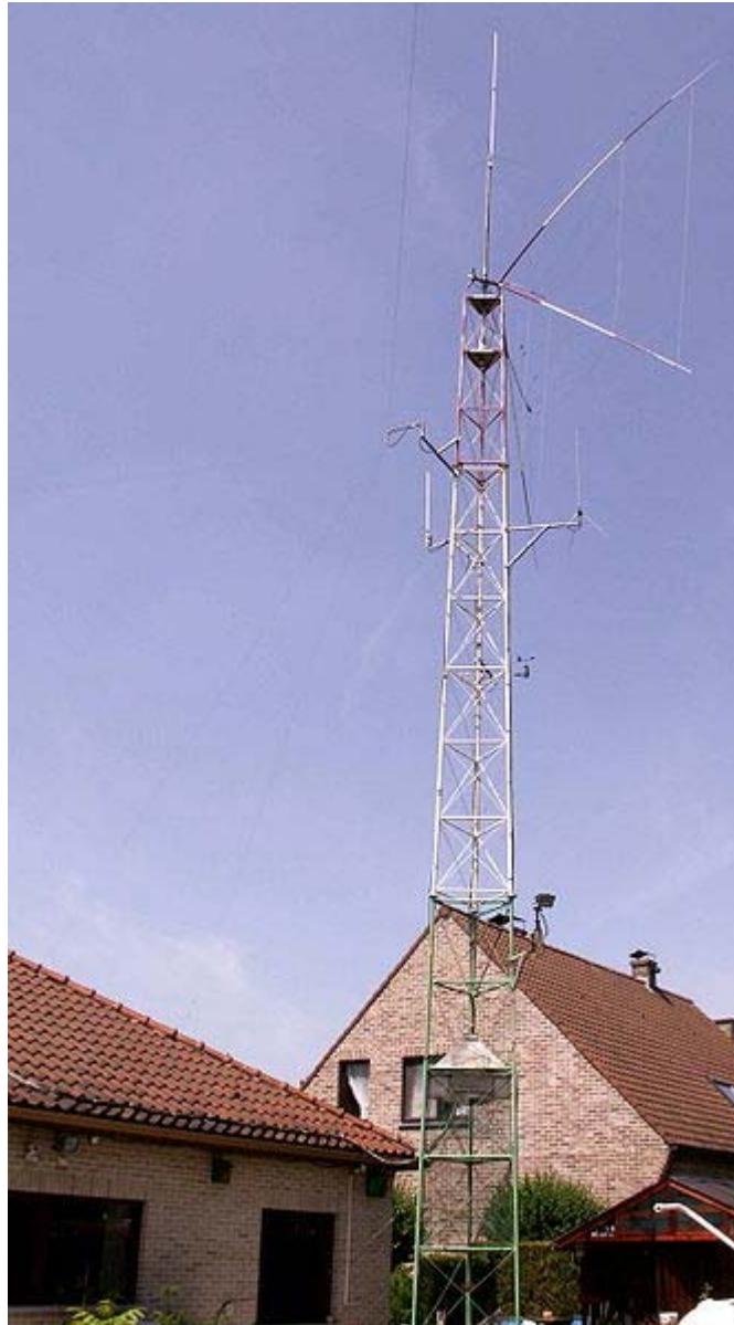
A radio amateur's do it yourself steel-lattice tower
