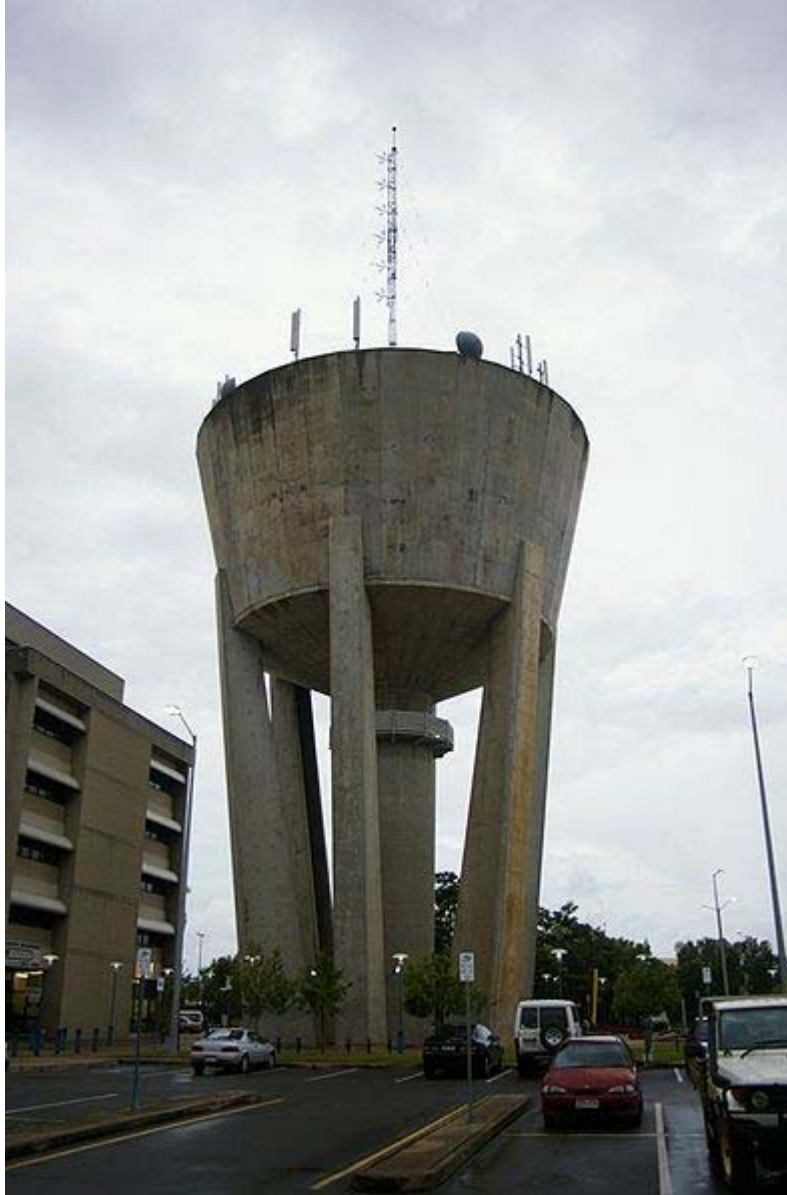
A water tower in Palmerston, Northern Territory with radio broadcasting and communications antennas.
