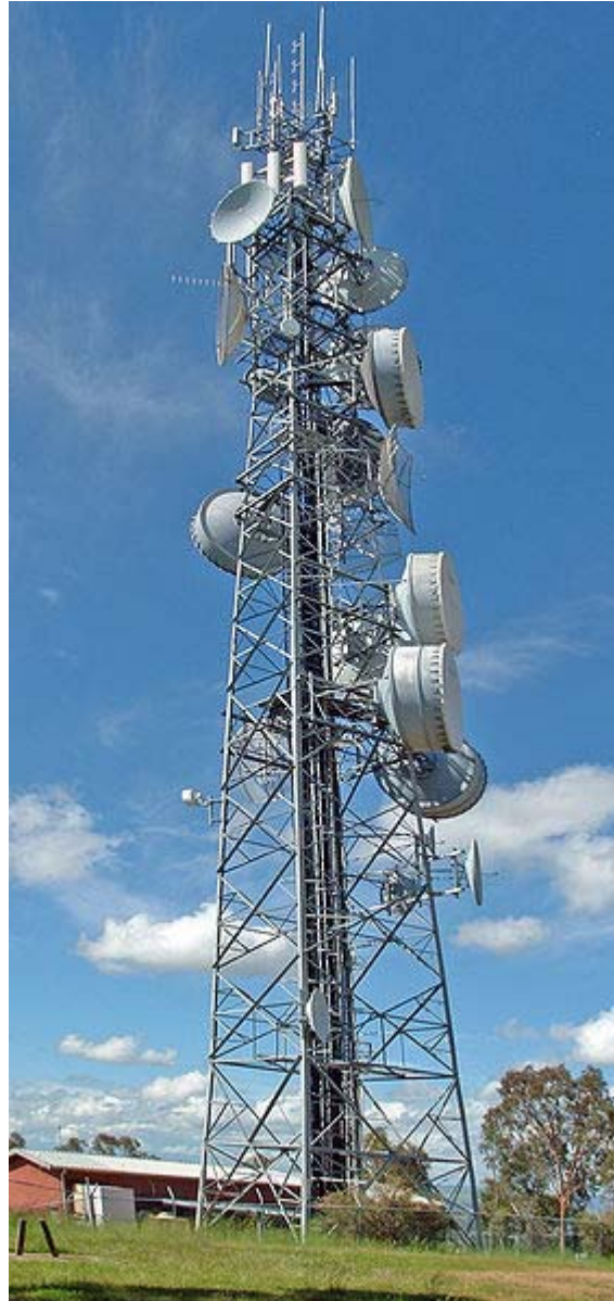
Steel lattice tower
