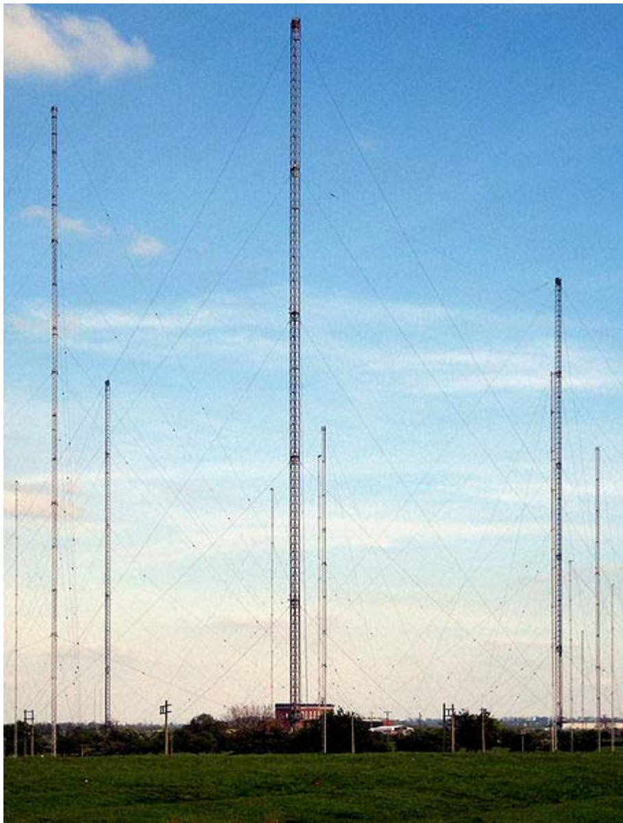
Masts of the Rugby VLF transmitter in England
