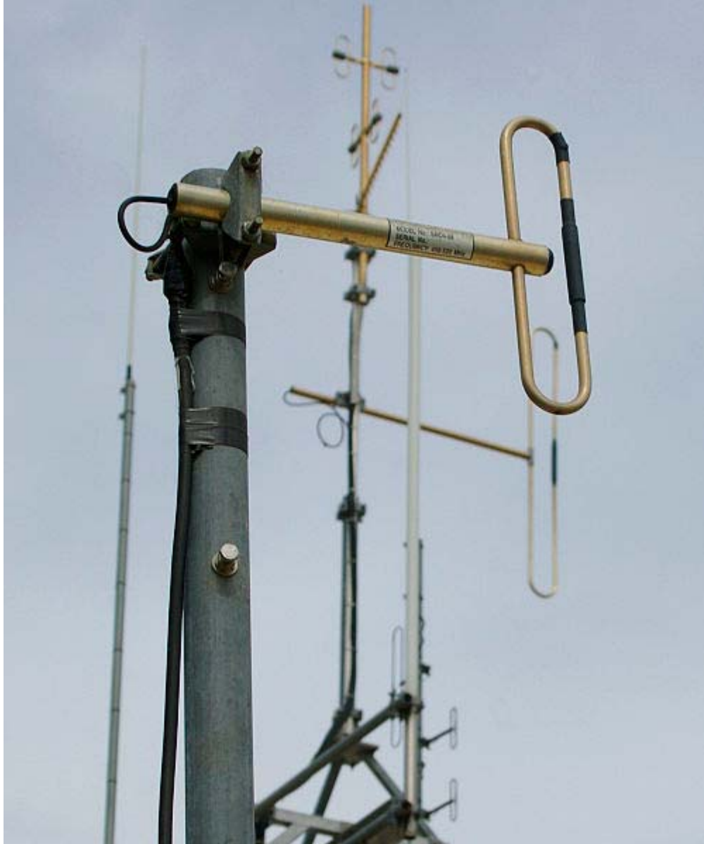
Folded dipole antenna
