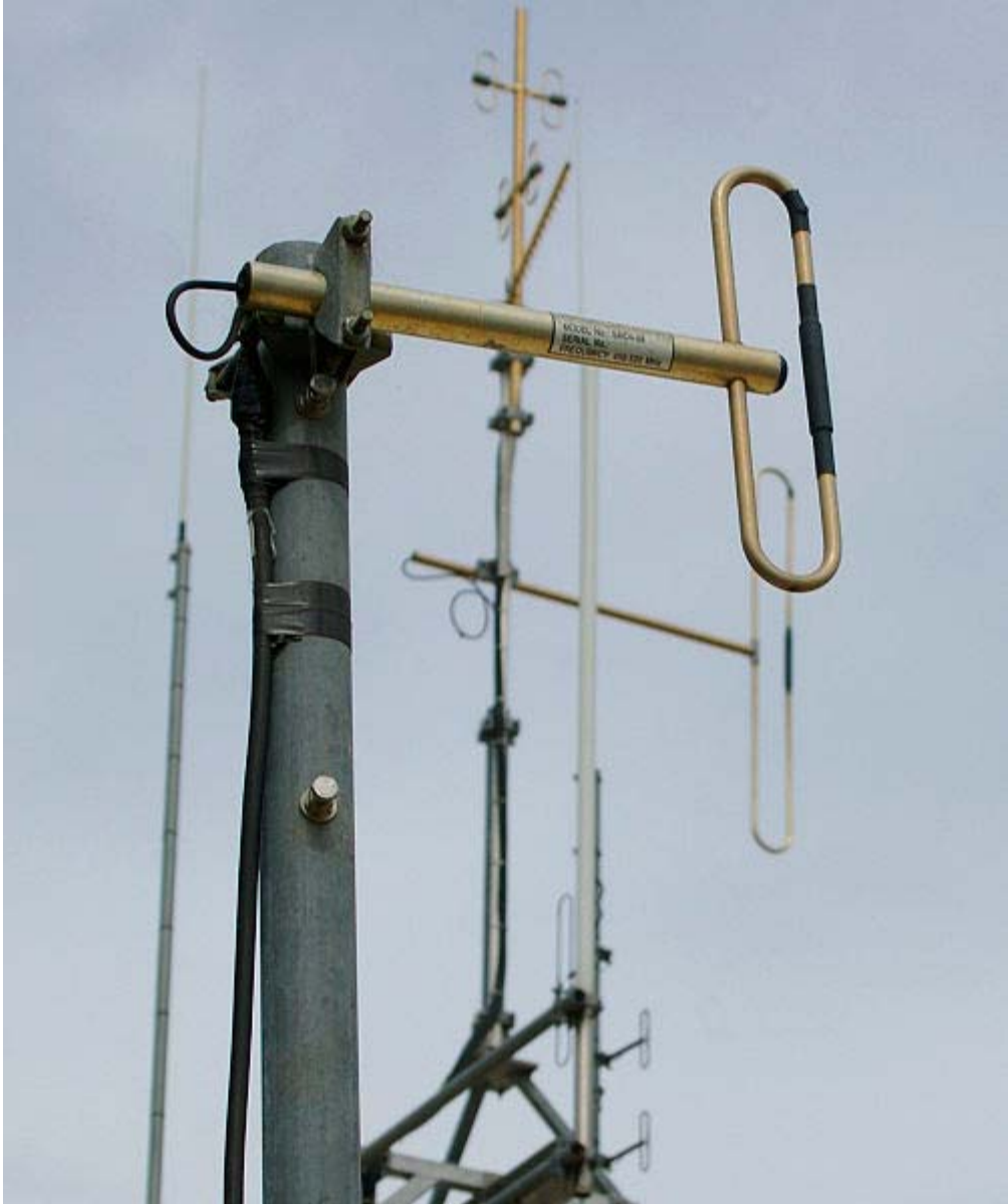
Folded dipole antenna
