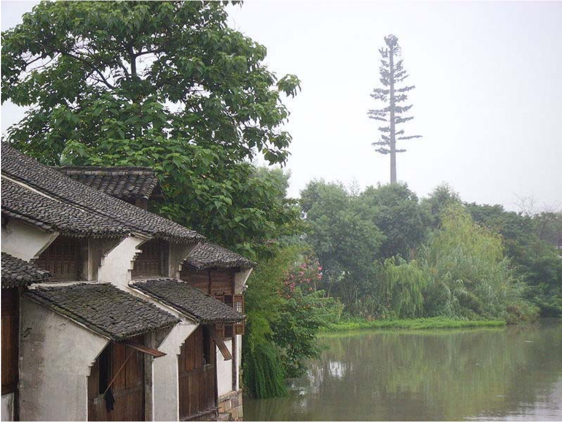
Communications tower, camouflaged as a slim tree
