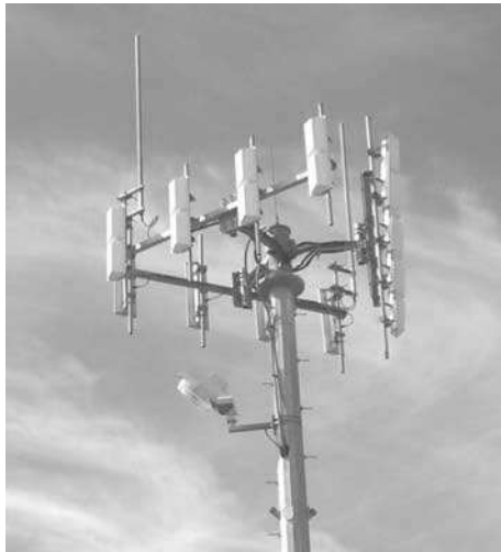
Figure 16.5 Sectorized base-station antenna.
