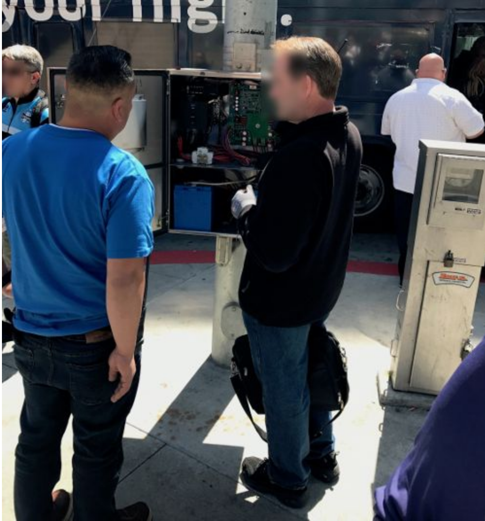
A San Francisco siren node being tested during the upgrade
