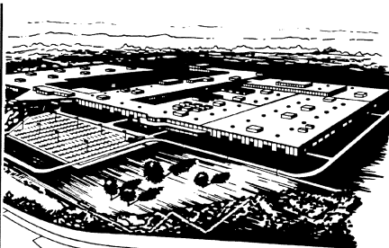
NISSAN MANUFACTURING FACILITY in Smyrna, Tennessee
