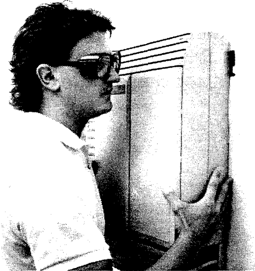
Figure 3.5 - Hanging the KSU
