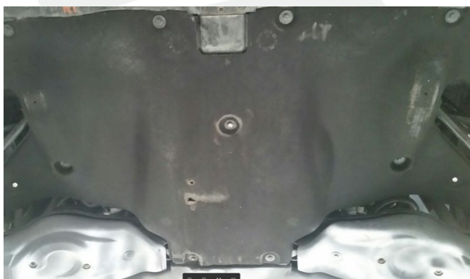
Figure 1 – Panel Abrasion; Not Covered
