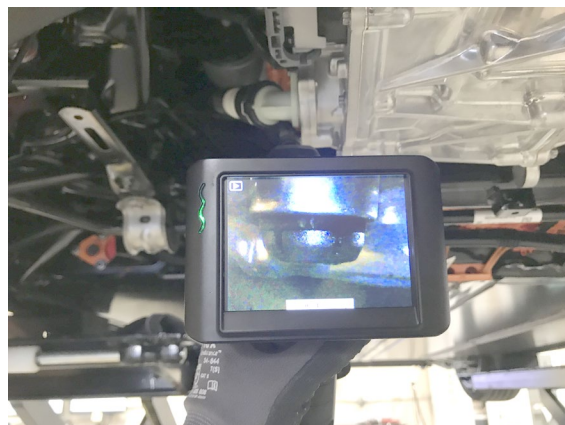
Figure 2 (Video scope view of breather installed)
