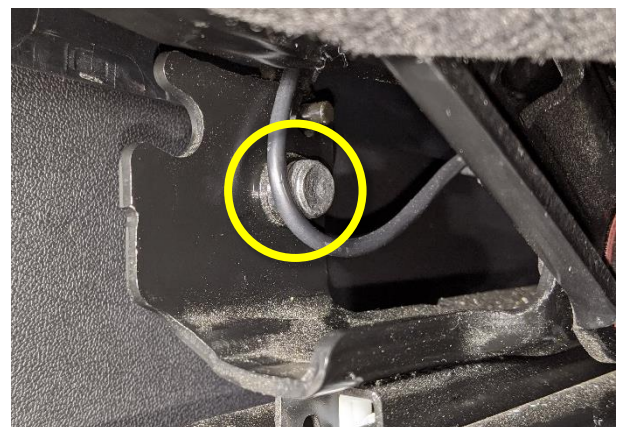
✗ Figure 12 – Harness around the seat recliner bolt
