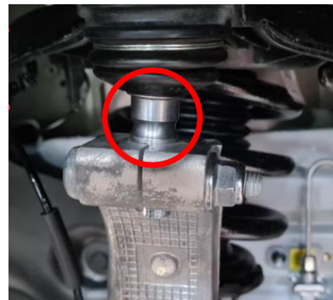
✗ Figure 4 – Joint not fully seated
