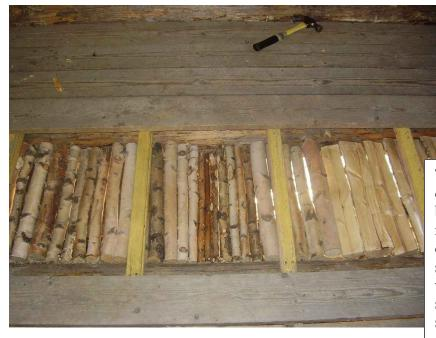
The floor upstairs is only 20 cm thick. The birches are representing the ceiling of the first floor. The space will be filled with paper or other stuff in order to absorb sounds.
