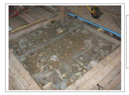
The finish of the foundation is made out of armored concrete. It holds the chimney, stove and oven- about 10 tons.
