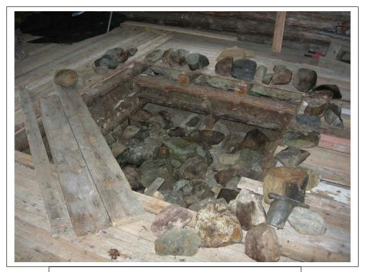
After leveling the floor downstairs, I had to raise the foundation through the floor. I made it from natural stones without concrete.
