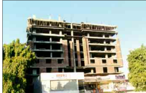
Fig 4.10: View of a typical RC complex
