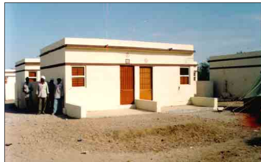
Fig 4.6: Typical cement block masonry house
