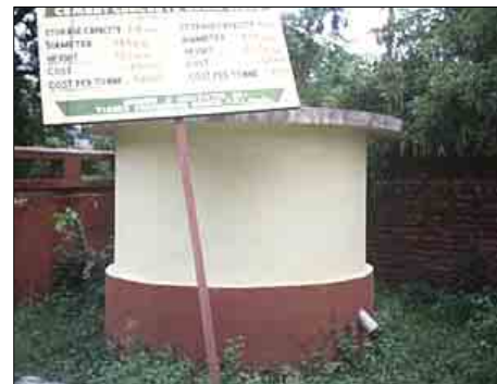
Fig 11.9: Bamboo-reinforced concrete silo
