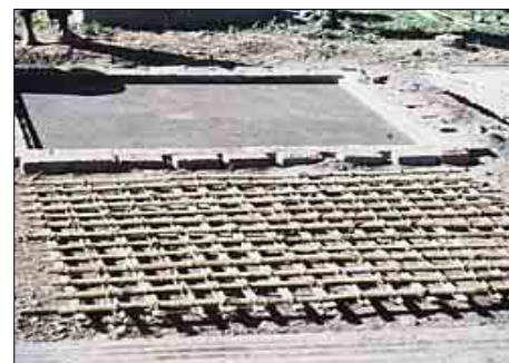
Fig 11.10: Bamboo reinforcement
