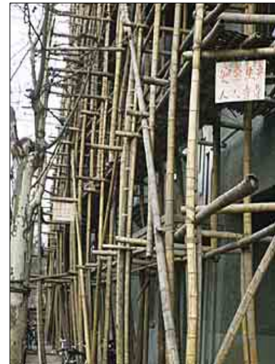
Fig 11.2: Bamboo scaffolding
