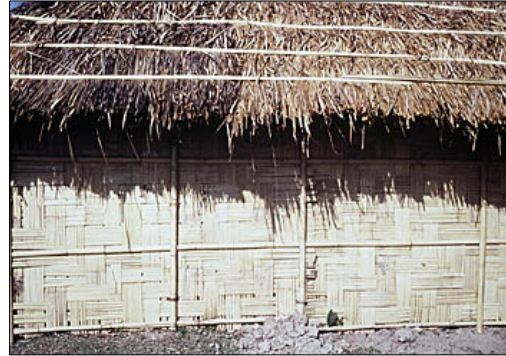
Fig 11.4: Bamboo mat wall
