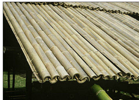
Fig 11.5: Bamboo tile roofing
