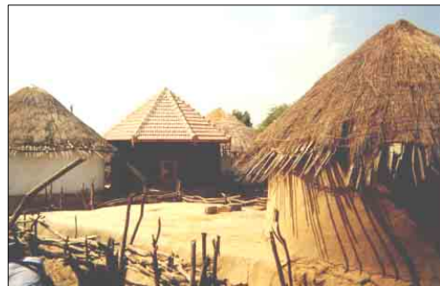
Fig 4.2: Bhongas that survived the earthquake
