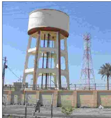
Fig 6.1: Examples of Good Performances during the Bhuj Earthquake
