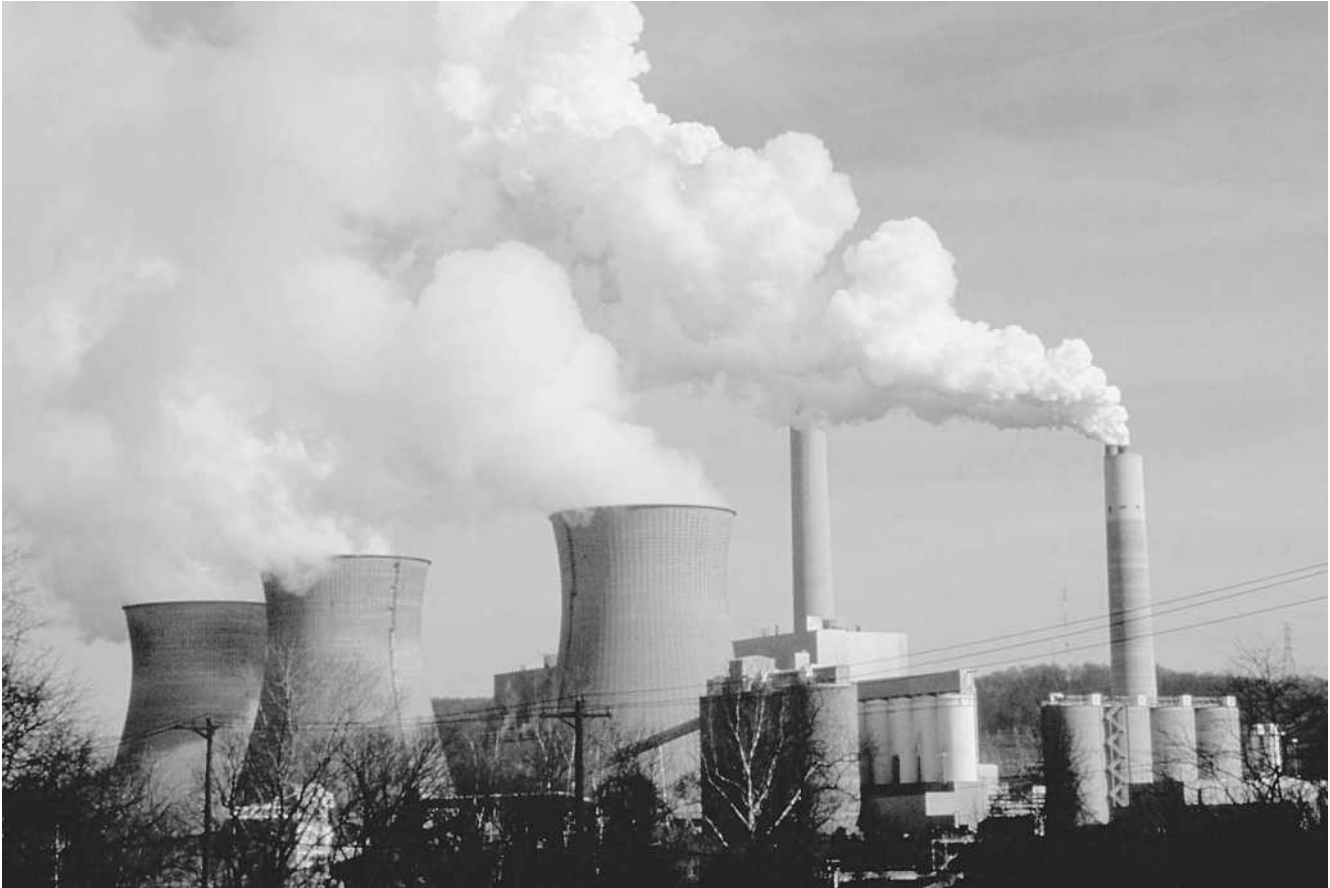
Electric power cogeneration site. (Greenpeace)
