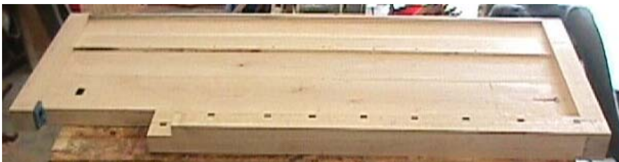
The bottom of the bench after the tool till tray was installed.
