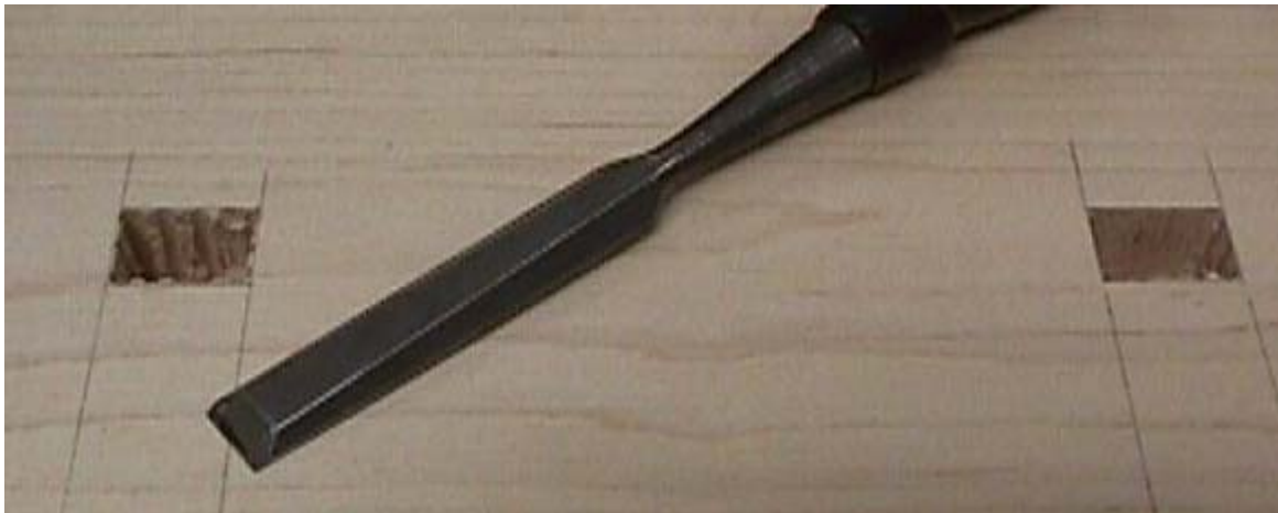
Cleaning up the holes with a chisel
