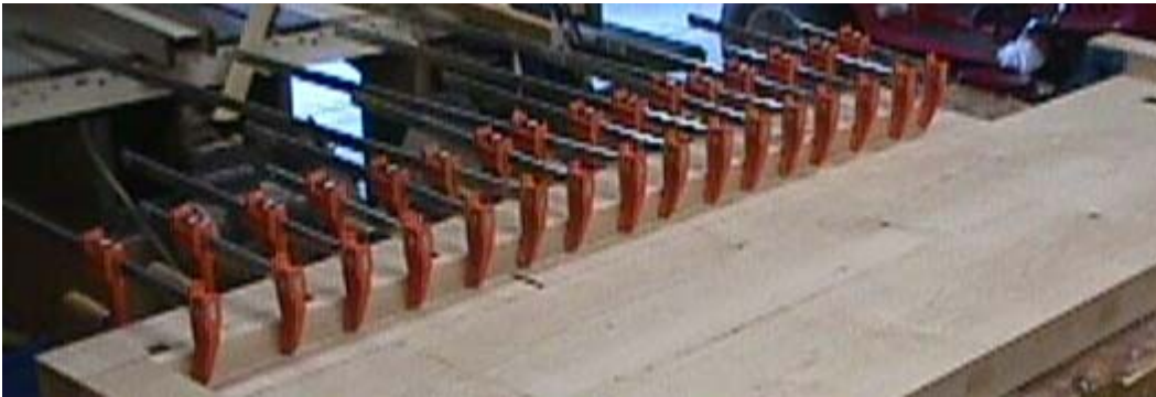
The Dog Hole Slot Cover being glued into place.
