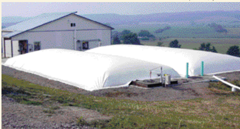
Photo 1. Beneath the polypropylene covers, waste is digested anaerobically. The dairy owners harvest the methane for energy production, which powers the operation. Excess energy is sold back to the area grid.
