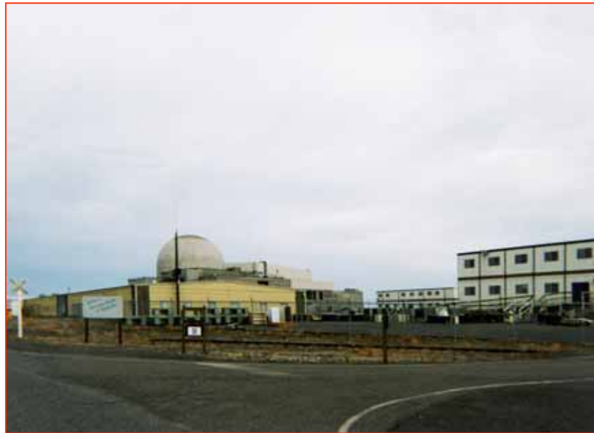
DOE Hanford site Richland, Washington
