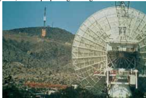
Fig. A.2.1. Microwave power transmission over 1.54km
