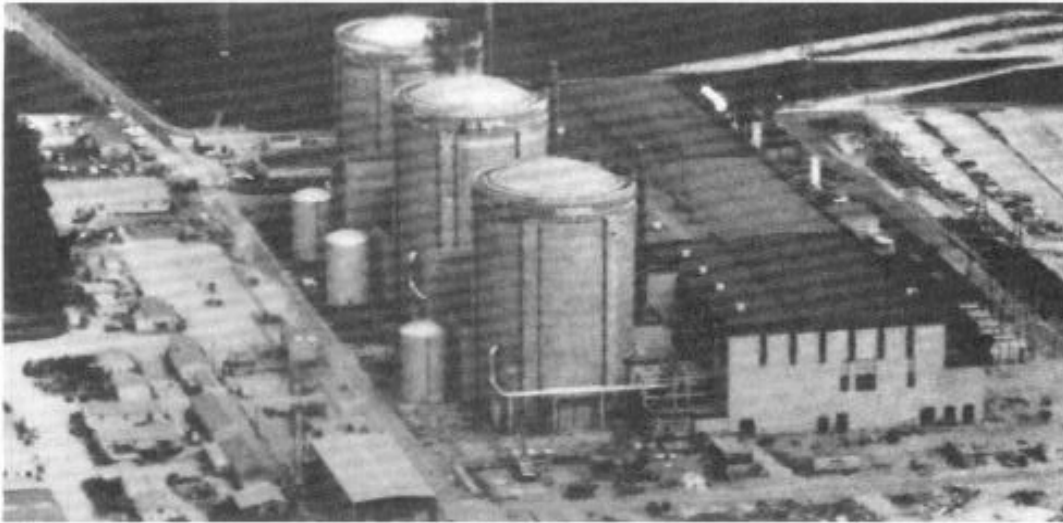
FIGURE 10.15 Oconee Nuclear Station of the Duke Power Co. (Courtesy of Babcock and Wilcox Co.)
