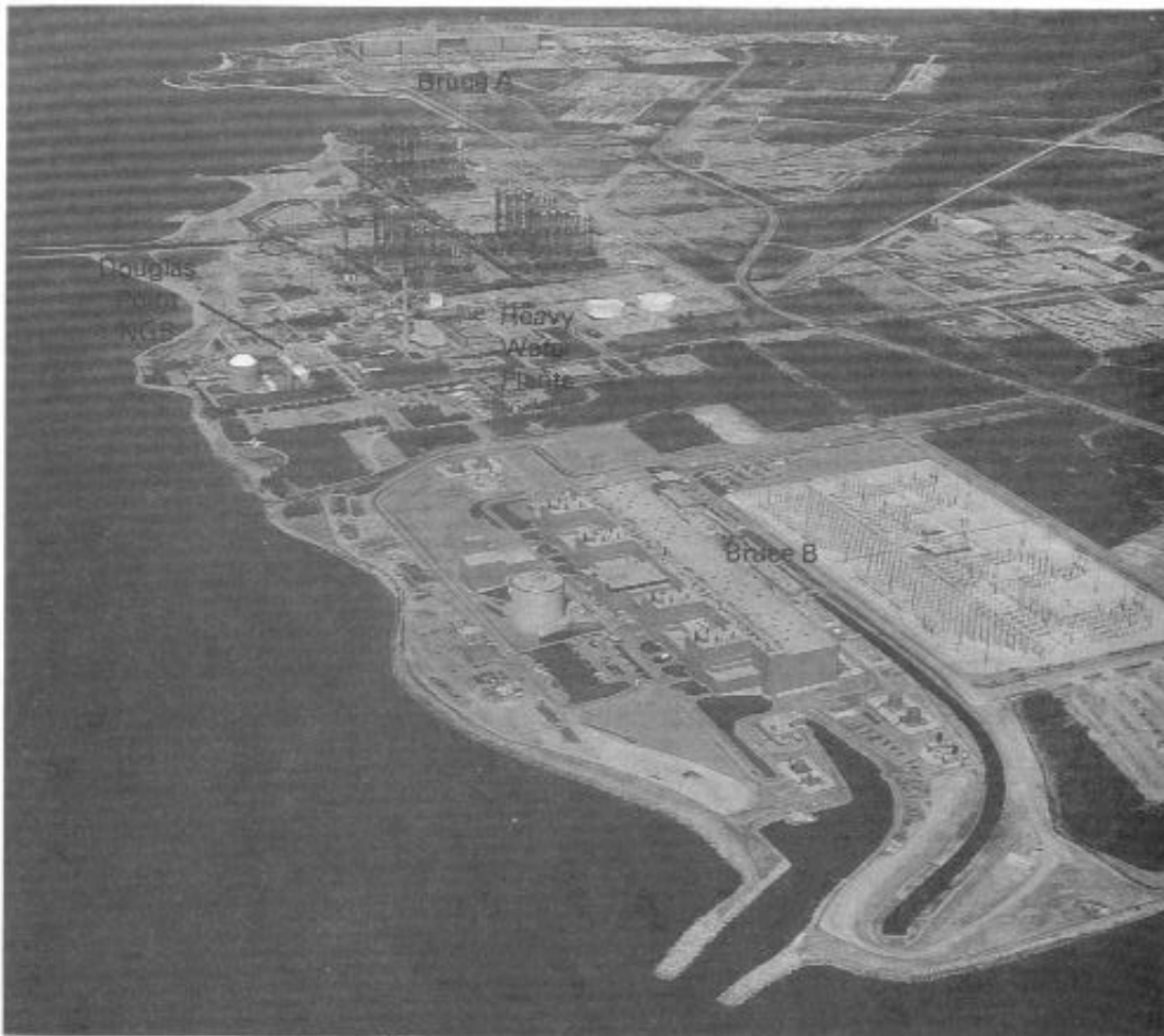
FIGURE 10.1 Bruce Nuclear Power Development in Western Ontario. Bruce A (3300 MW) is at top, and Bruce B (3660 MW) is in the foreground. The Douglas Point Nuclear Station is at far left, and the Bruce heavy-water plants are just to the right. (Courtesy of Ontario Hydro, Toronto, Canada.)
