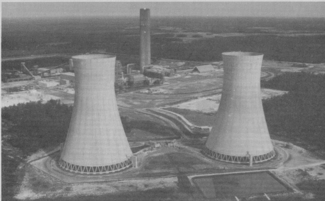
FIGURE 4.9 Hyperbolic natural-draft cooling towers. (Courtesy of the Marley Cooling Tower Co.)
