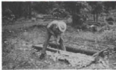
Fig. D.17. Hewing flat sides on a pole with a sharp ax.
