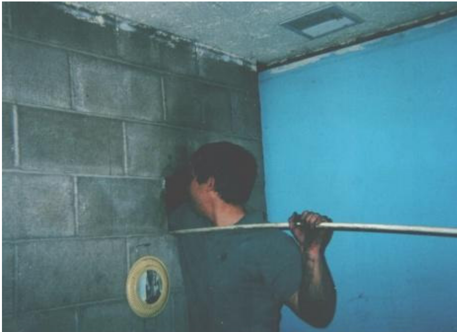
Guide the brush up the chimney while pushing with the shaft.
