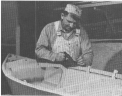
Fig. 4 Cut and screw on the gunwale fillers and cockpit corner knees, as shown in the plans, then glue and screw these in place. Cut deck stringers and fasten them, then bevel
