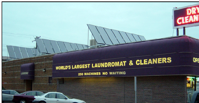
Twentyfour flat-plate 4' x 10' Solar Collectors
