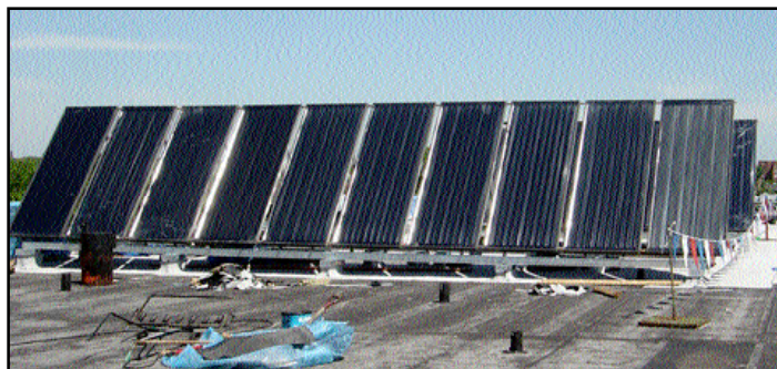
Twentyfour flat-plate 4' x 10' Solar Collectors
