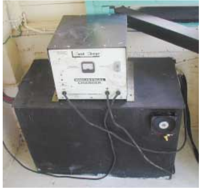
The AC charger, used for grid backup, sits atop the vented battery box that holds four Trojan L-16Hs.
