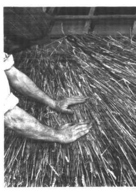
The needle is now inserted in the new position which is the edge of the yealm just laid. A levering motion is used to force the work tightly together.
