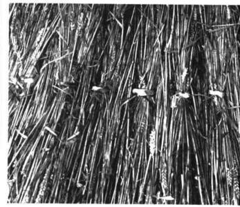
There is, however, an alternative method by which a course can be secured. This is by twisting a straw 'bond' or 'scud' which is sparred down in the same fashion.
