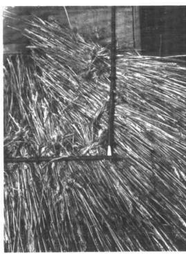
Turning to the gable (or barge) the bottles are laid in the same way, each one overhanging the barge-board by half its length. The sway is started by forcing the large end, which has been tapered for the purpose, behind the sway holding the eaves.
