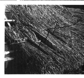
From this angle it is possible to see the position of the sway holding the second and third courses, where it overlaps the vertical sway which holds the bargebottles.
