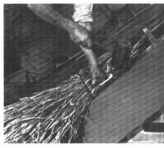
The position of the spar is indicated in relation to the barge-board which is seen immediately below.
