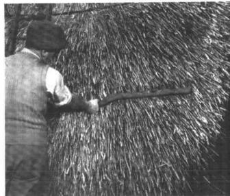
When a section of the roof has been covered in, the side-rake is used with a combined beating and combing action.
