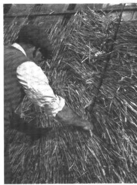
Before any courses are laid, a thin layer of straw is spread as a lining course over the battens. Although it is not a necessary requirement, it does have the effect of making the roof neat and tidy when seen from the inside. It should not however be confused with back-filling as used with other materials.
