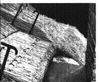
Thatching is now continued by tying in the wadds to form a short eave behind the chimney. A tilting fillet is fixed at the appropriate distance from the first batten to which the wadds are tied. The lead may be carried up as far as this batten if desired.
