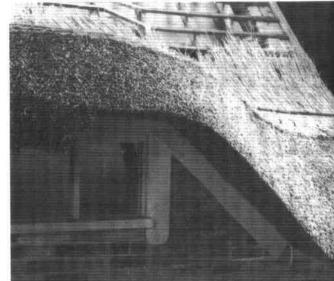
Cutting the eaves is usually carried out at a later stage of the work, unless of course light is obscured or windows are prevented from being opened. Starting in the centre of the window the eaves-hook is used, working from left to right.
