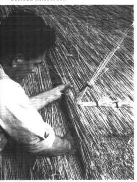
It is most important that a good join is made each time a bunch is laid. This is done by raising the edge of the course with the left hand and then working the nearest reed to it well down to the bottom of the course.
