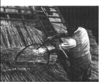
Before the courses are started it is suggested that a layer of back-filling is applied. This will prevent the tops of the courses from penetrating between the batten, and also give a neater finish inside.
