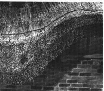
The same process occurs on the left-hand side of the window where, after the browcourse has been laid, the second course is started from the point of gradation.
