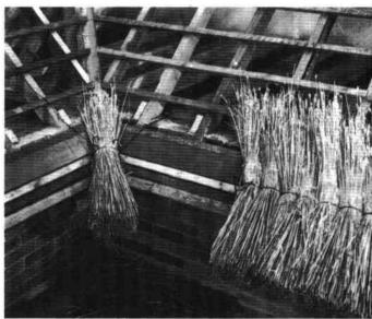
A firm solid corner has been obtained by turning the reed towards the cutting-line.
