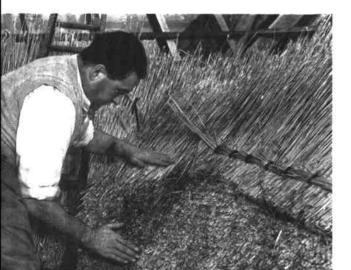
The first course is carried through and the hazel sway is fixed. The joint in the valley angle is made by inserting one sway below the other.
