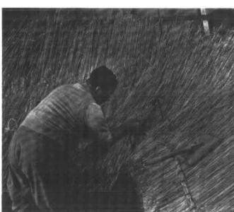
At this stage a packing layer may be laid within the area indicated by the two needles. The object of this is to take the sharp angle out of the valley and to increase the pitch of the courses.
