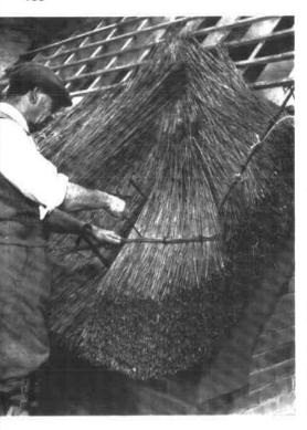
A light fixing method is now used. A small quantity of reed is placed across the course which is firmly pinned down with iron hooks to the tight reed beneath. This is known as a temporary sway and is later removed.
