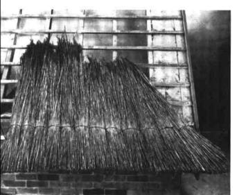
Closer inspection of the tie shows how the cord passes twice round the batten before being wrapped twice round itself. Because of its tightness, the cord is prevented from slipping and the bunch is securely held.
