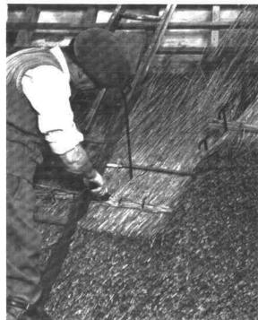
As previously stated the reed in the angle of the valley lies with less pitch than the reed on either side. To counteract this, and thereby to give the water equal discharge, a long coarse bunch is opened and laid with the butt-ends uppermost, and with the lower ends just covering the sway. This will be fixed with the succeeding course and may be repeated at intervals as required.
