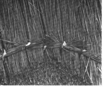
Long thatching-hooks are used to secure the temporary sway, but with certain thatchers the spar or brotch is still preferred for this purpose. The method is a survival of the days preceding the introduction of the iron hook, when stitching with grass rope or hedge briar, and later with treated cord, were the only methods of binding employed.
