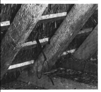
The needle is then inserted into the reed at a suitable point, where it appears immediately above the batten. The cord is removed from the eye of the needle by the assistant who works from inside. The needle is then withdrawn to the outside.
