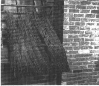
It next becomes necessary to fit the lead gutter behind the chimney. Raised in the centre, the gutter sheds the water in both directions. The sides of the lead are dressed on to the reed and the stepped-flashing on either side.
