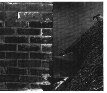
A closer view behind the chimney shows the neat, tidy finish obtained, and it is unlikely that a gutter of this construction will become blocked by falling leaves or other rubbish. There is also room for a man to stand, which in itself facilitates subsequent work on the roof.
