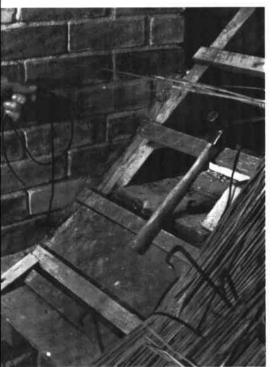
If an obstruction such as an eaves-chimney is encountered, a break in the eaves-line is made and courses must be terminated. To ensure a strong finish next to the chimney, the staple and cord method can be used.
