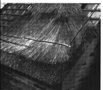
Brow-course fixed with hazel sway. Hooks are driven into every rafter and the portion of temporary reed sway is removed in preparation for laying the next course.
