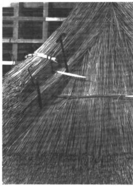
The next full course is once again started by setting the hip-bunches. It is recommended that this is done by laying two half-courses, the first being fastened before the second half is laid. By this method a very much stronger hip angle will result and the face of the finished coating will be tighter and closer together.
