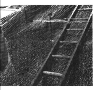
Laying the brow-course to the window calls for extra care if a good eaves-line is to result. Selected bunches are merged together with the left hand to avoid gaps and spaces appearing after dressing.
