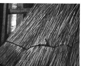
A very useful method by which the final bunch can be tied when filling in the gap, is illustrated. A loop is made in the end of the string which holds the corner bunch.
