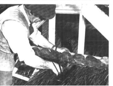
The sedge apron is laid by taking a good double handful of sedge, and after turning down the long ends at the top to make a tight bunch, it is worked firmly under the sill. The needle is inserted beside each bunch as it is laid and is used to force each section tightly together. The whole of this layer is fastened down with a 'scud' or 'bond' which consists of several pieces of sedge twisted together rope fashion, and sparred down into the course of reed underneath.
