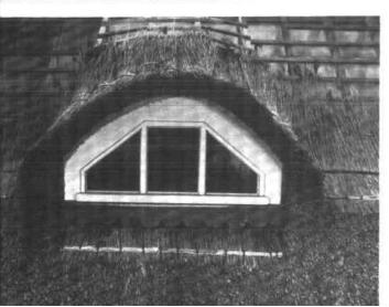
These eaves-bunches are carried to the centre of the window, and at this stage the eaves are neatly dressed into line to conform with the required shape. It will be noted too that the sway is cut off and the 'tying in' method used. This is really a matter of preference, but it is suggested that with each bunch secured to the batten, there is less likelihood of any movement or slipping taking place at this point, where the reed is subject to greater wind pressure.
