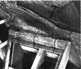
A gable dormer is the type of abutment which has a ridge to it, and makes its junction with the main roof at a point below the ridge-line. It follows therefore that very careful treatment is required at the junction to make a sound finish.
