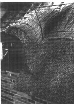
Special care is needed when the eaves-bunch is laid on the angle of the window.
