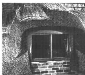
Fixing the eaves-bunches is now completed and the hazel sway is secured in readiness for the next course.
