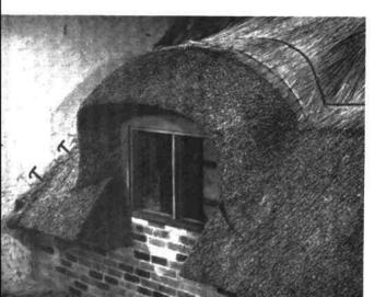
The first full course over the window is completed and is ready for the sway to be fixed. A close inspection is worth while in order to see how the join is made.
