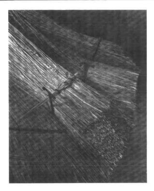
The brow-course may be laid next, but it is suggested that the work will be greatly assisted if the hip-bunches are laid first on both angles as shown in the illustration.
