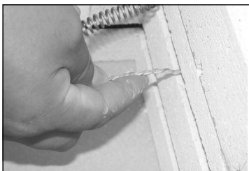
Inserting the new element into the firebrick hole.
