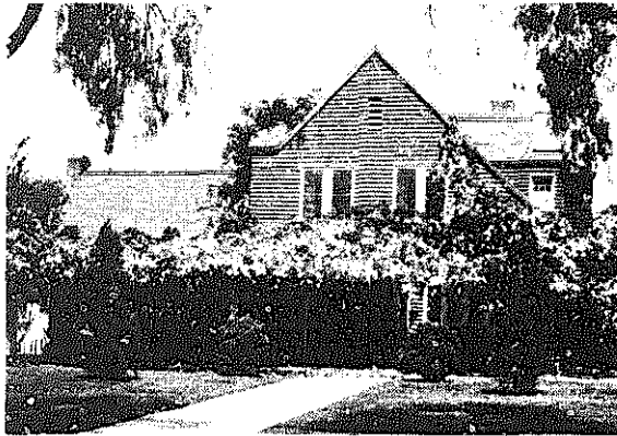
A Glendale, California, residence equipped with a Walker solar heater (seen at upper right corner of roof).
