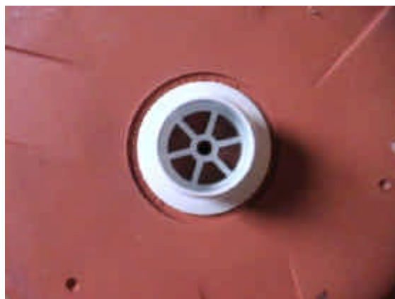
A perfect fit. See notes about sealing this with plumbers jointing compound later on. Extremely important.
