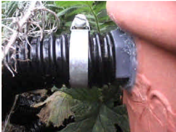
This is the 40mm outlet and piping which I used later on.... (notice the jointing compound to seal the join). This pipe feeds off into a large hole carefully drilled into the back of the terracotta urn, which sits at the top of the waterfall.
