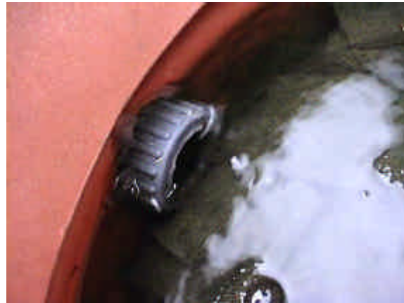
This larger 40mm outlet has much better capacity to let the water flow out.
