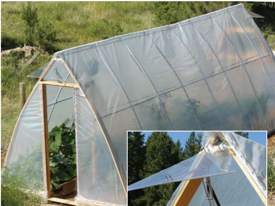
Gothic greenhouse with heavy-duty conduit, automatic-venting mechanisms on the tops of the end walls and a much simpler end wall structure and door.
