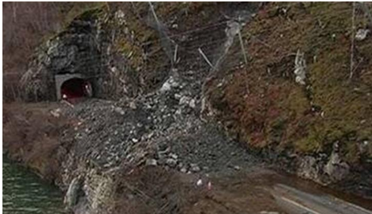
This landslide is an effective roadblock, but was it natural, or deliberate?
