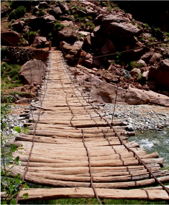
Rope and stick bridges can be made with widely-spaced rungs, to use less sticks, if wood is scarce.
