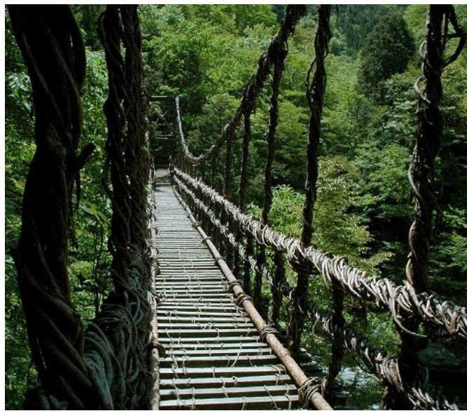
Large vine and stick bridges have thick suspension cables, made from many vines twisted together.
