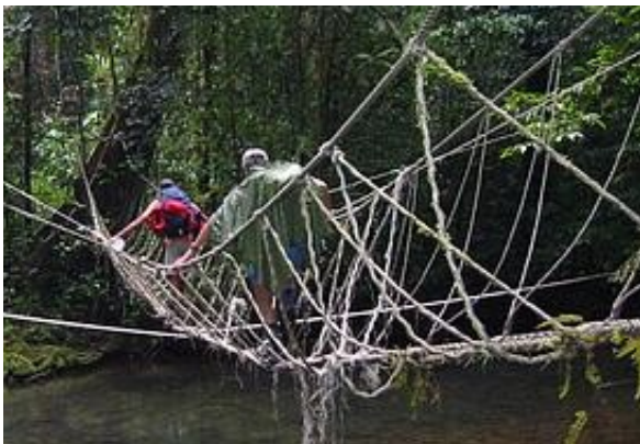
Guy ropes can be tied to the bridge on either side, and are used to reduce the notorious sway of rope bridges. Using extra rope (or vines) on the hand lines makes crossing a rope bridge safer.
