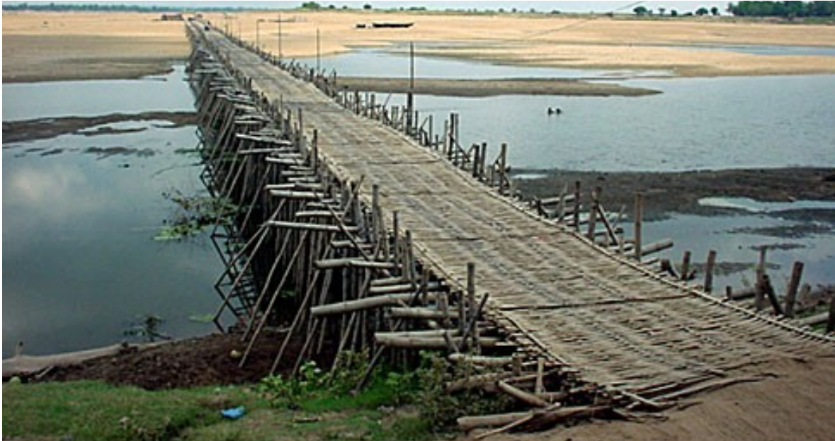
This large bamboo bridge lets vehicles transport garden produce to a local market.
