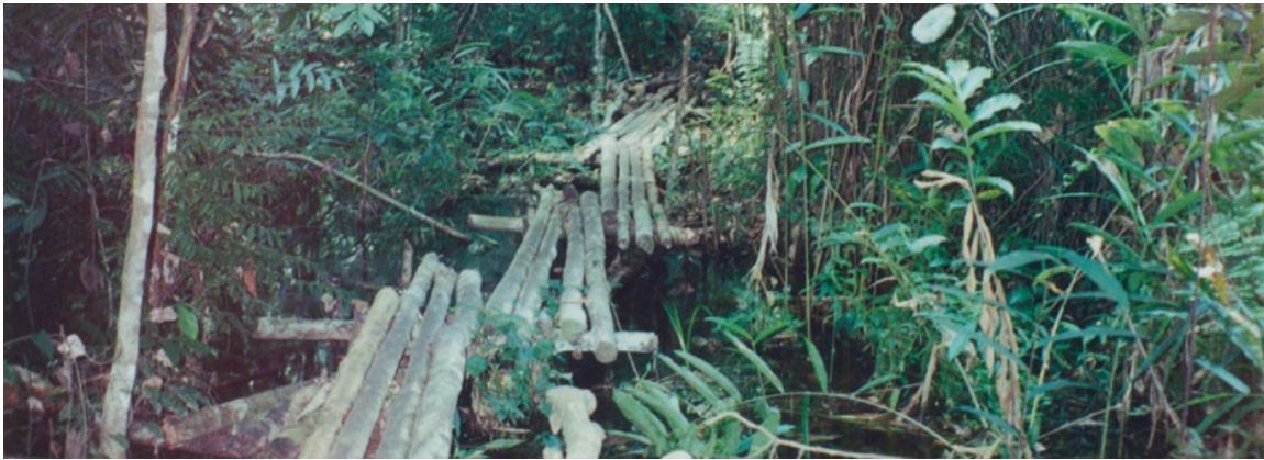
In swampy areas, a series of bridges can be used to span wide stretches of marshy ground.
