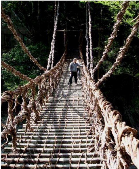
Large vine and stick bridges have thick suspension cables, made from many vines twisted together.
