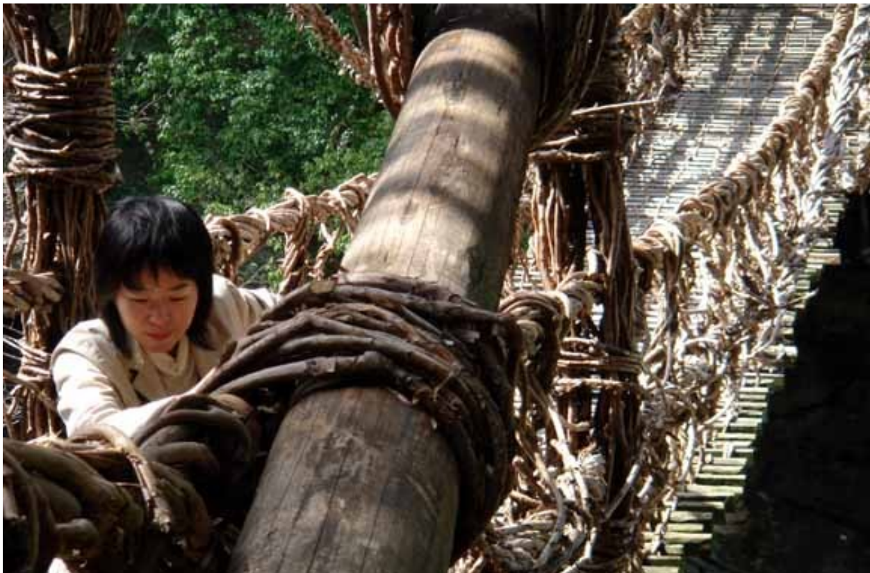
Vines are woven while green, and secured with hitches; tying knots in vines will make them split.
