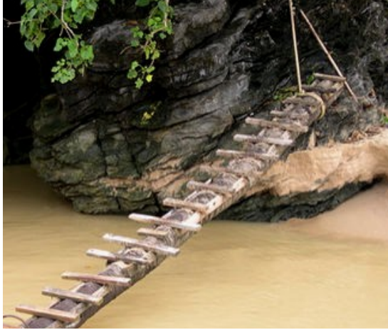
Other bridge types; these one-log and two-log bridges are made with widely-spaced plank steps.
