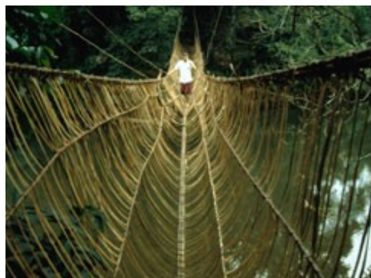
Guy ropes can be tied to the bridge on either side, and are used to reduce the notorious sway of rope bridges. Using extra rope (or vines) on the hand lines makes crossing a rope bridge safer.
