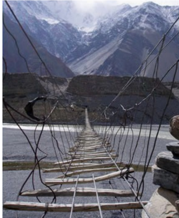
Rope and stick bridges can be made with widely-spaced rungs, to use less sticks, if wood is scarce.
