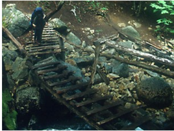
Other bridge types; these one-log and two-log bridges are made with widely-spaced plank steps.
