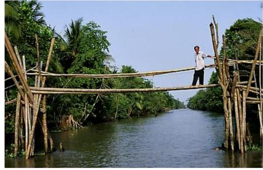
Simple bamboo balancing bridges, with handrails.
