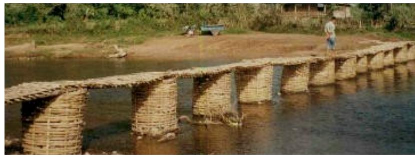
Bamboo pylon bridge (pylons are filled with rocks, for stability).
