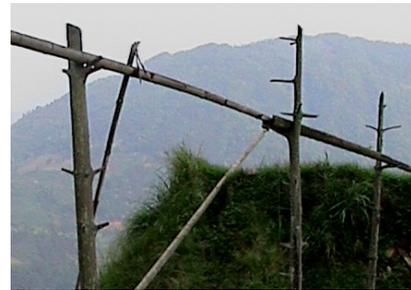
Bamboo pipes that carry water downhill, and support poles (made from small trees).
